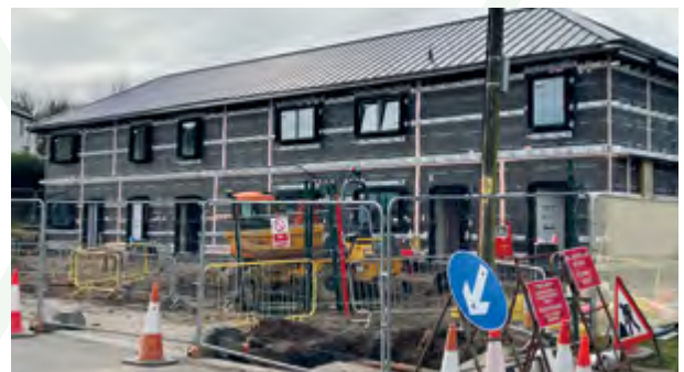
Affordable housing development at Treceyndd (Caerphilly Homes)
