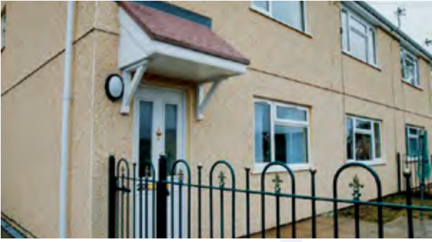
Homes at Rowan Place, Rhymney after external improvements
