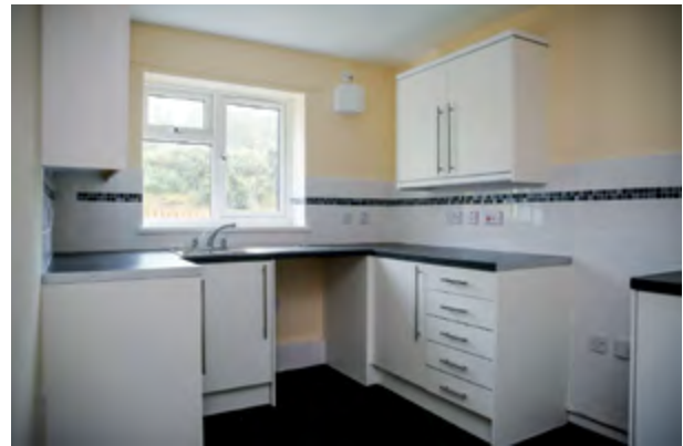
Kitchen replacement under Welsh Housing Quality Standard programme (Caerphilly Homes)
