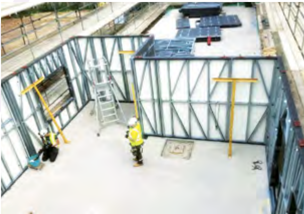
Construction of innovative steel frame system at Trecenydd (Caerphilly Homes)
