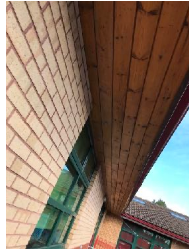
Tight fitting soffit boards
