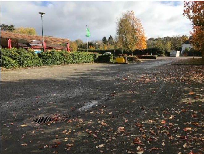
Tarmac & vegetation to south east
