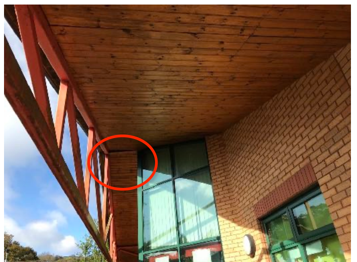
Overhang of south facing gable
