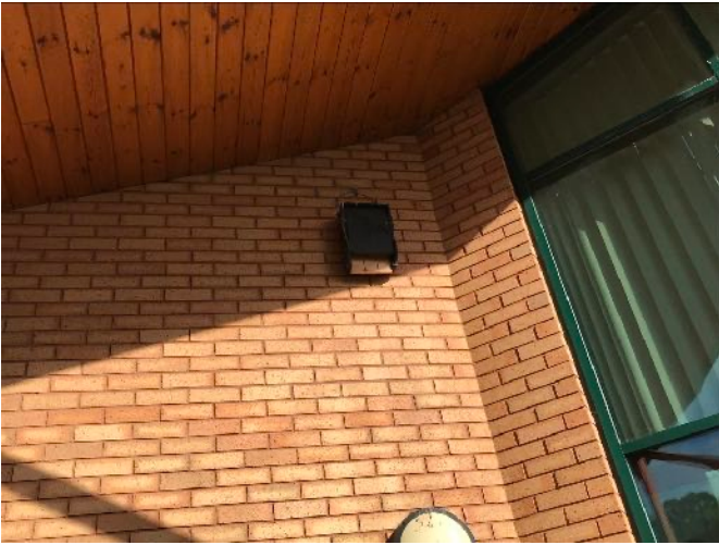
Bat box on south facing gable wall
