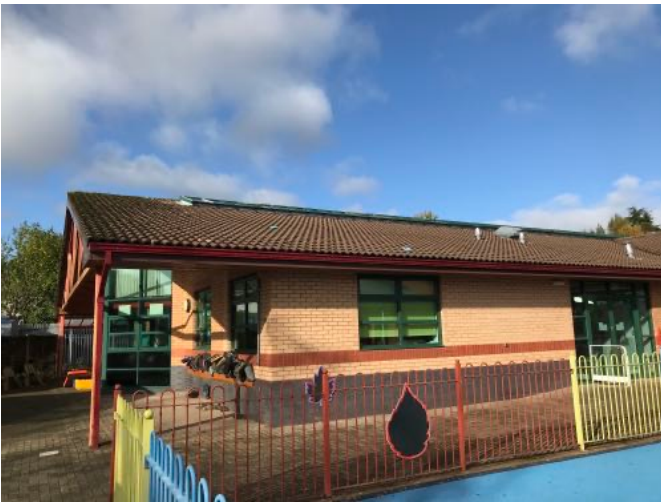
East facing pitch of southern extension
