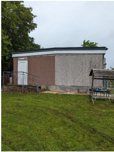
Figure 23 - Southern aspect of the nursery building.
