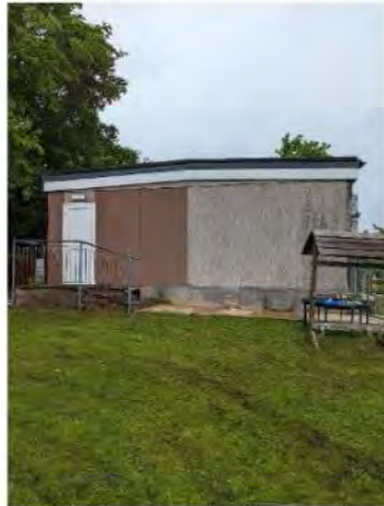
Figure 23 – Southern aspect of the nursery building.
