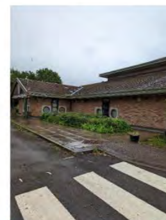
Figure 19 - Western aspect of the building (area of roof to be affected by the works).
