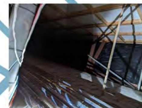
Figure 20 - Visible loft space at the west of the building.
