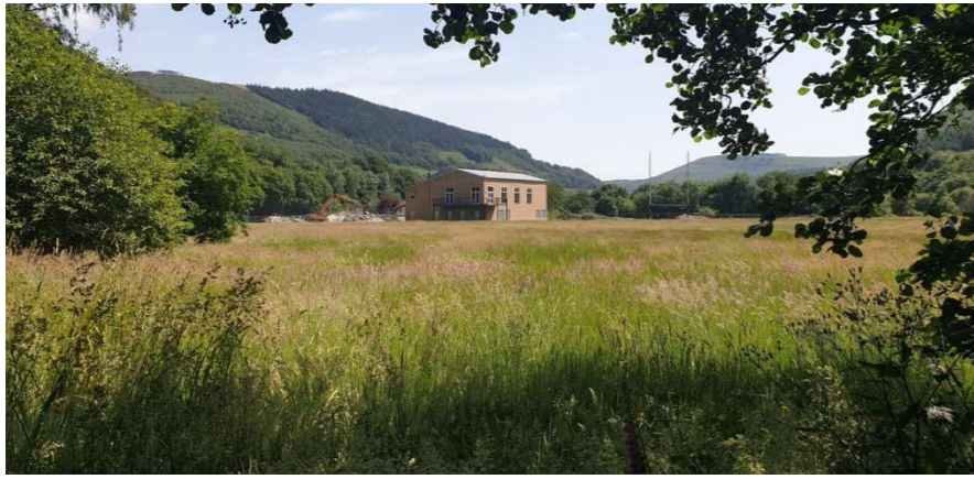
View 7: South East to Performing Arts - Block C
